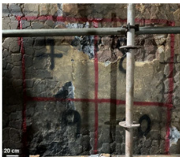
Fig. 3: Refractory lining spalling due to thermal shock damage.
