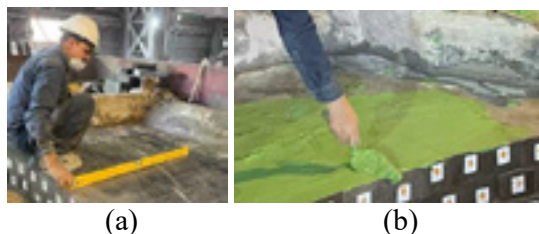
Fig. 3 (a) check the flatness, (b) mortar patching.
