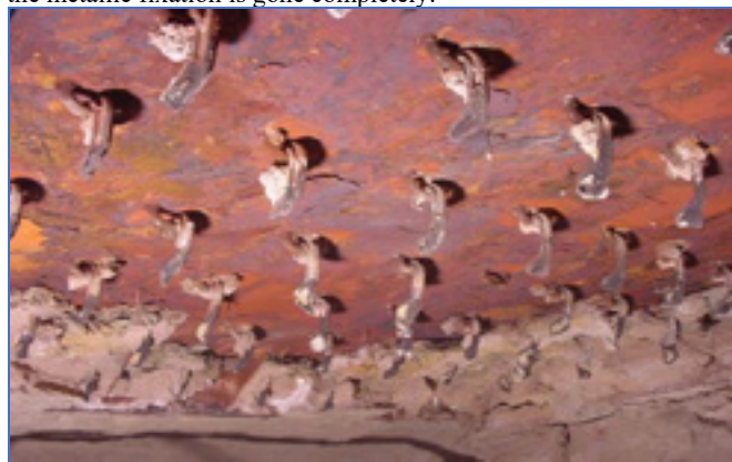
Pic. 1: Corroded anchors, roof section
