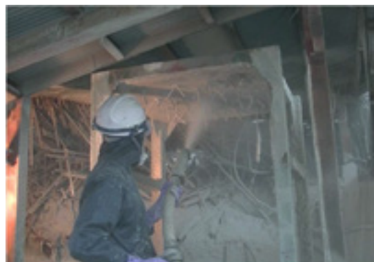
Fig.1 Appearance of dry-gunning test.
