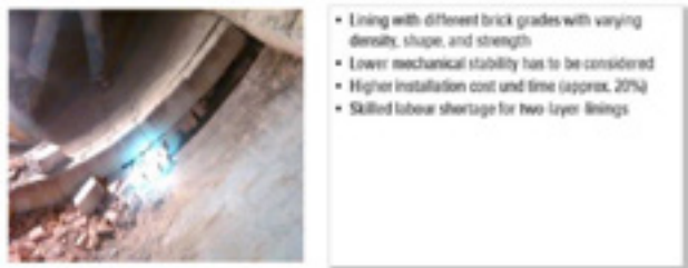
Fig. 10: Mechanical destruction of a two-layer lining
