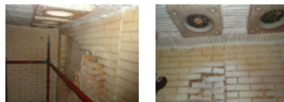
Fig. 3: Deteriorated refractory around burners.
