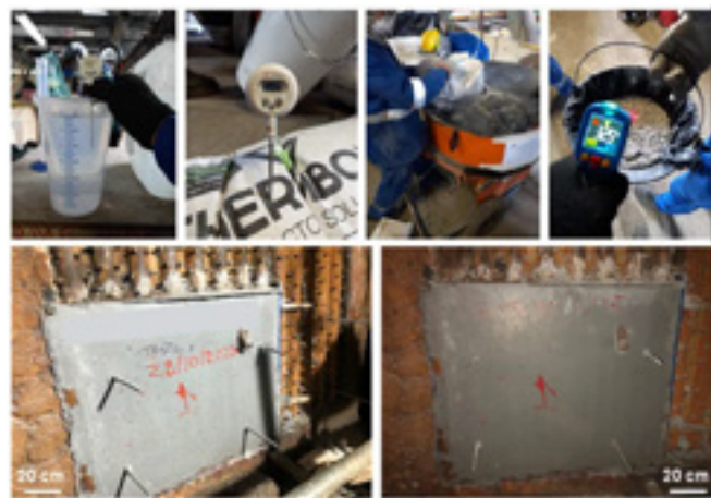
Fig. 8: Applications of the self-flowing phos-bond castable: next to the burners (lower furnace) and close to second air nozzles.
