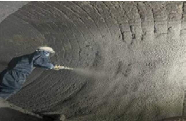
Fig. 1. Shotcrete repair in torpedo ladle car
