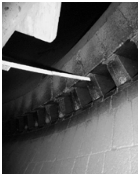
Picture 3. Gas inlet area 2014 shifting of the lining
